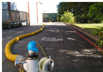
Soil vapor extraction testing at the Savings Square Shopping Center. (Source: EPA)
