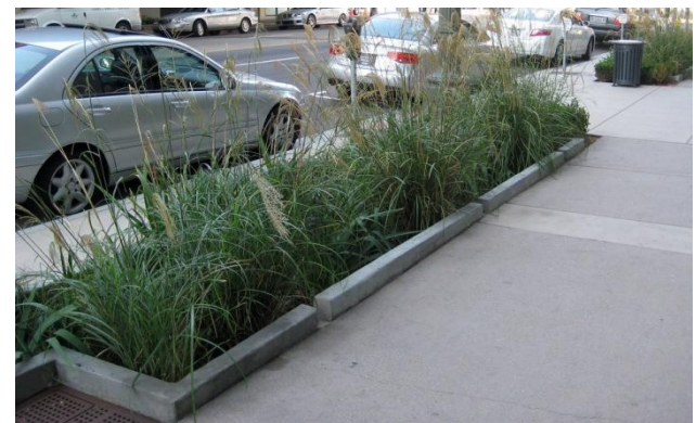
Stormwater Planters, Los Angeles, CA Source: Mia Lehrer + Associates
