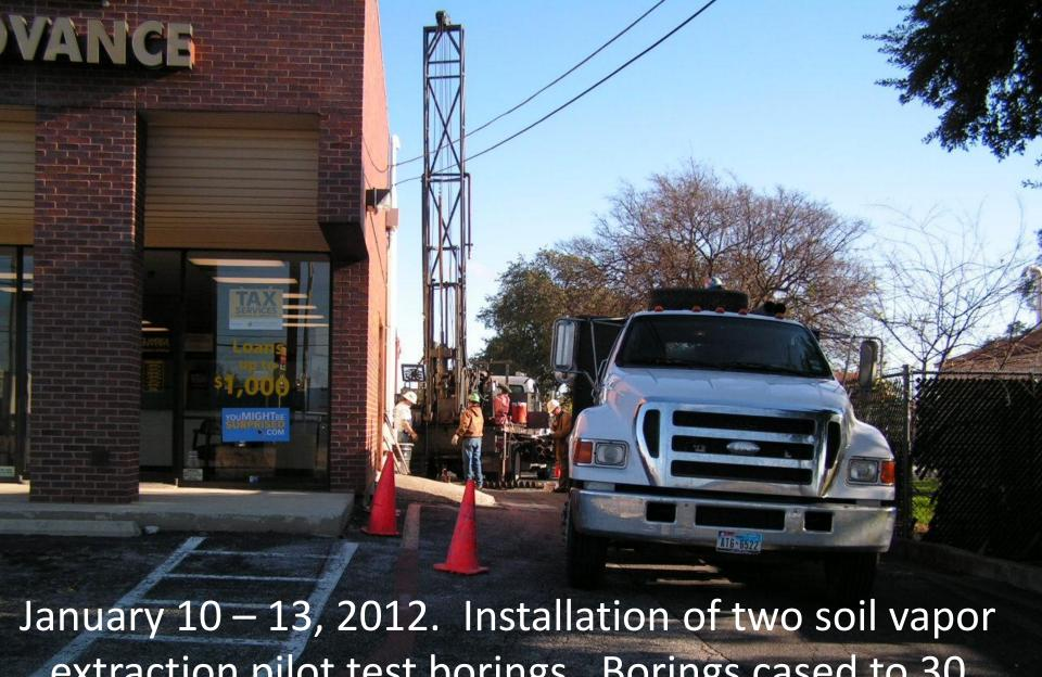
extraction pilot test borings. Borings cased to 30 feet, open hole from 30 to 50 feet.
